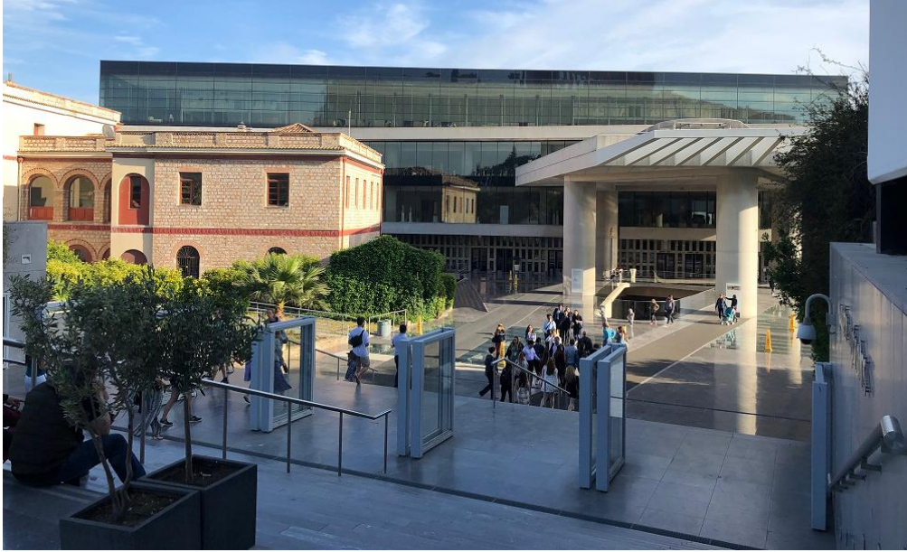
3.5 South elevation, NAM, Athens, May 2019. Note lack of vertical structural evidence between the three main floors of the building while the thickness of the floor slabs is exaggerated. Note also the three different treatments of each floor - vertical concrete screen, vertical glass, horizontal glass, moving upward from grade.
