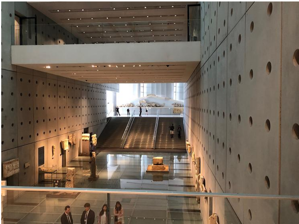
3.7 Westward view from mezzanine, NAM, May 2019. Note screened glazed floor creating the illusion of a floating stairway, hanging in time and space. Note also the perforated (i.e., screen-like) wall treatment recalling that even the stair treads were screened glass.
