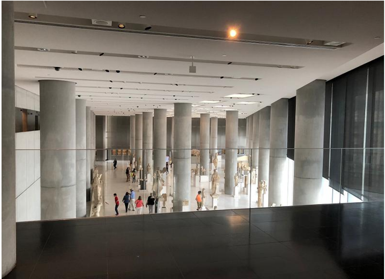
3.12 View from mezzanine to second floor hall of columns, NAM, May 2019. Note the number, spacing, and size of the circular, drum-formed, concrete columns.
