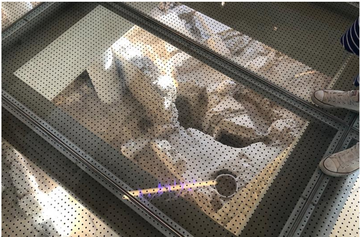
3.8 Screened glazing at ground floor also used at stair treads, NAM, May 2019. Note untouchable artifacts beneath floor plane.
