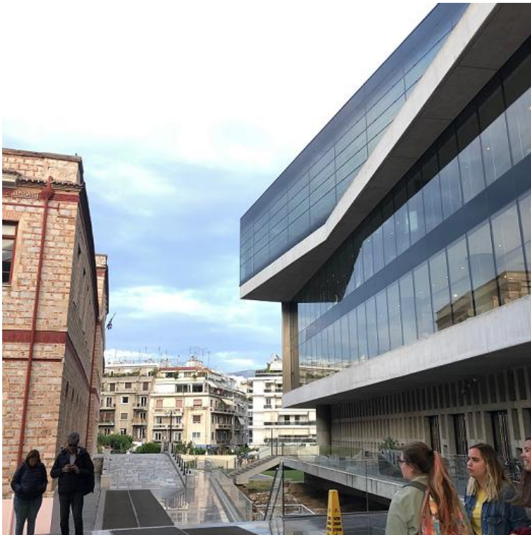
3.6 Partial south elevation of NAM, Athens, looking westward, May 2019. Note 1) skewed floor plate, top floor; 2) vertically oriented concrete wall screen at first floor, vertically oriented glass at second floor, horizontally oriented glazing at torqued top floor; and, 3) that the lowest floor plane appears to float over grade.
