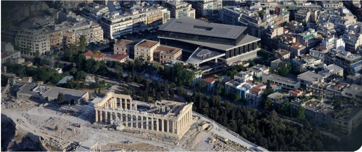
3.2 The New Acropolis Museum, Athens, Bernard Tschumi Architect, 2009. Southward view from the Acropolis illustrating the torqued top floor apparently cranked into parallel with the Parthenon.
