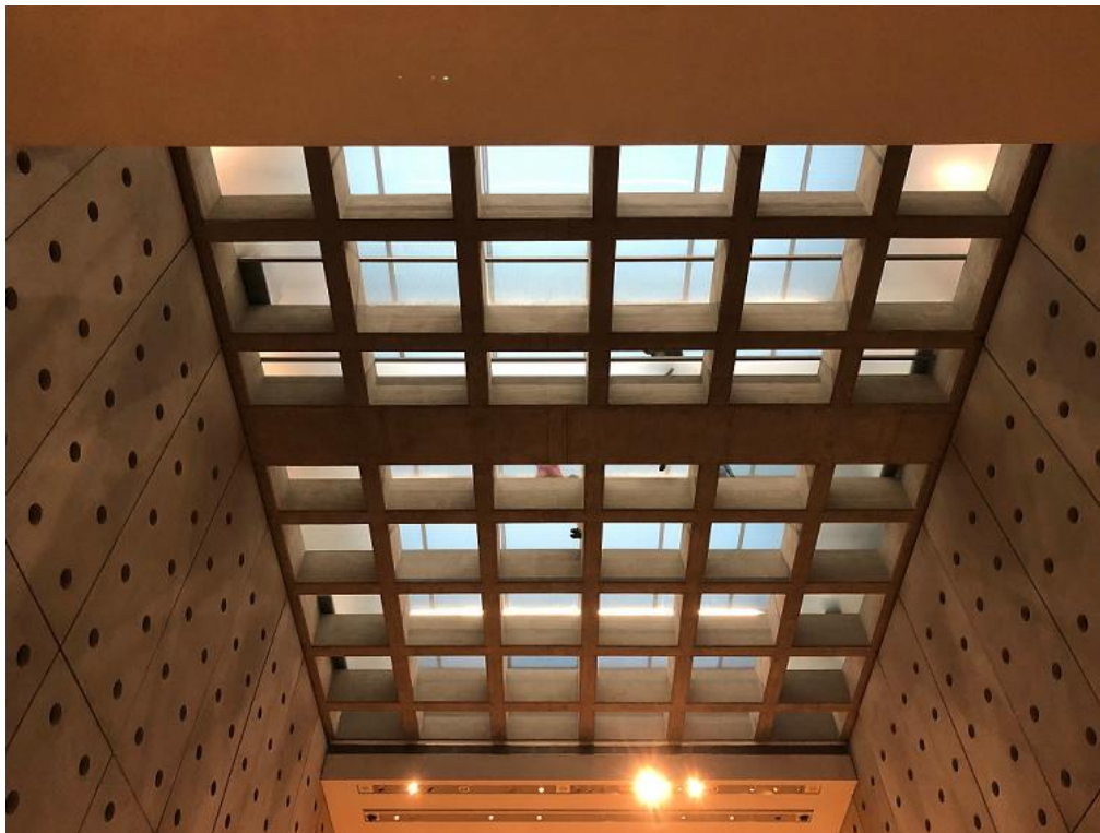
3.9 View of deeply coffered ceiling, NAM, May 2019. Such ceilings were also typical of classical spaces though this one was intentionally designed without the typical layers of ornamental moulding associated with more classical precedents.
